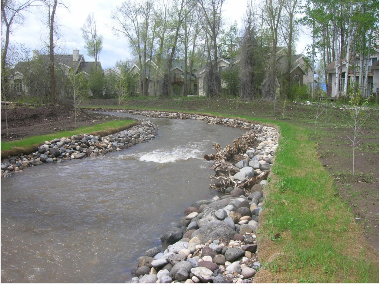
Restored side channel
